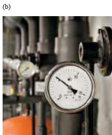
12.9 (a) A Bourdon pressure gauge. When the pressure inside the flexible tube increases, the tube straightens out a little, deflecting the attached pointer. (b) This Bourdon-type pressure gauge is connected to a high-pressure gas line. The gauge pressure shown is just over 5 bars (1 bar = 10^5 Pa).
